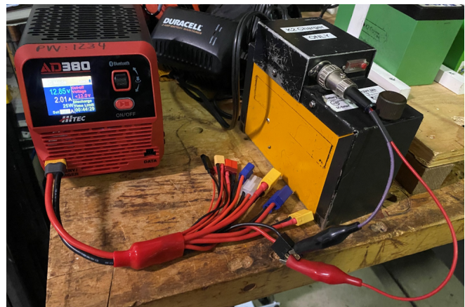
Figure I. Discharge Testing Repaired Battery
